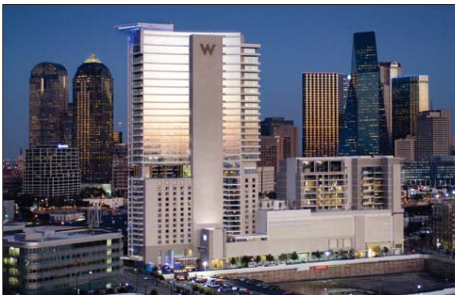
Hillwood Development Corporation's Victory Park project has helped to revamp the landscape near downtown Dallas.
